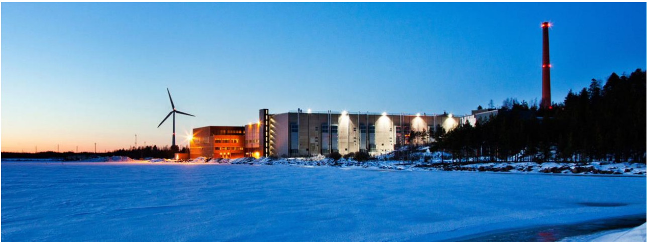
Fig. 14. Google's Data Centre in Hamina, Finland, sited near the Bay of Finland for cooling purposes. The race for renewable energy is already on between the big tech companies [31] (photo: Google, cropped)
